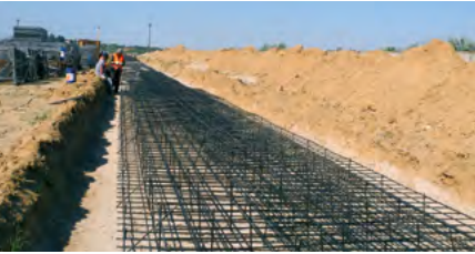
Warehouse complex, Mykolaiv, Ukraine
